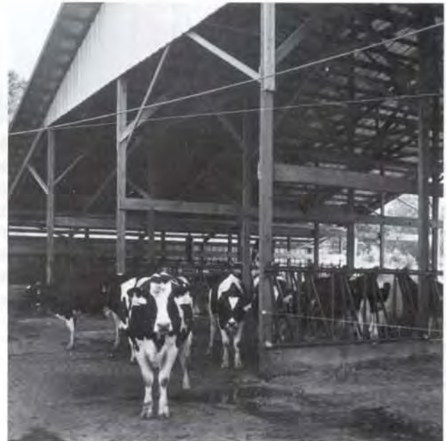
Design facilities for maximum air flow.
